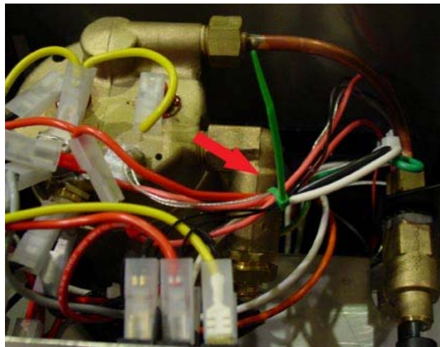
Figure 24. Tie up the cables.
